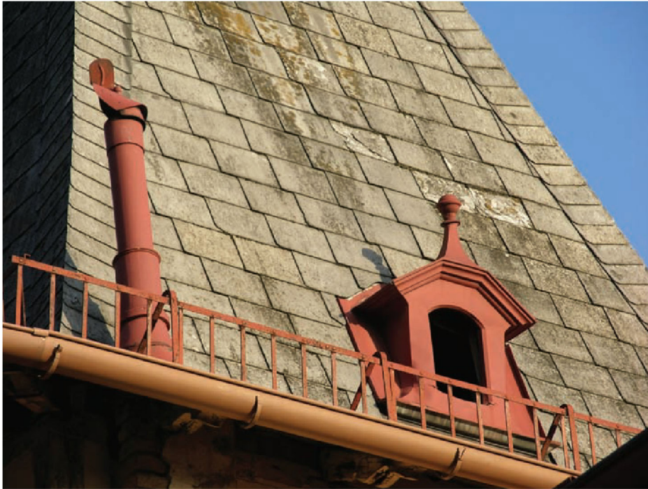
A roof covered with asbestos cement tiles
